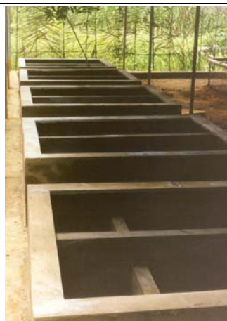
Above: Ten aquatic tanks were constructed within a new 6 x 14 m 2 quarantine cage. Each cement tank includes a small terrestrial section where turtles may bask or spend time on land. The new quarantine facilities were built with support from Rotterdam Zoo. Right center: Heosemys grandis and Hieremys annandalii enclosures under construction (with support from WWF Japan). Lower right: The new quarantine cage after completion. Plastic tubs hold aquatic turtles recently received from the trade.
