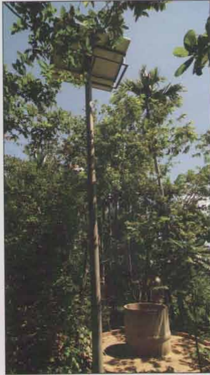
Left: The nesting beach on the Sre Ambel River is guarded 24 hours per day during the nesting and hatching seasons. Pictured here is the guard coming to shore to transport biologists to the nesting beach. Middle: New solar panels will serve to power pumps for moving water from the well to water storage tanks, where the water will be gravity fed into the headstarting facility. Right: Three wild caught River Terrapins ( Batagur affinis ), some of the last of their kind in Indochina, held in captivity for over 10 years at a facility in Koh Kong. These turtles represent valuable genetic additions to the captive program. Major improvements at the Sre Ambel facility are required before these turtles can be moved.
